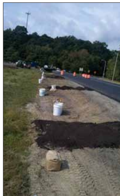
Research on roadside stabilization applications of biosolids compost and other fertilizers (photo courtesy of Dr. Rebecca Brown)
