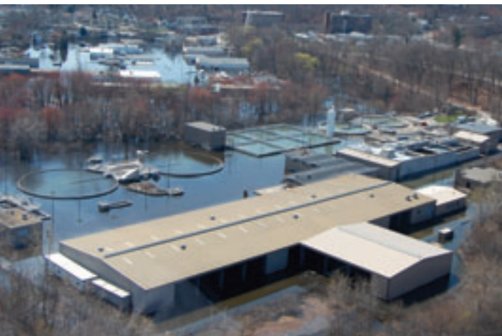
The West Warwick, Rhode Island biosolids composting facility closed last year after its site was flooded and the equipment ruined.
