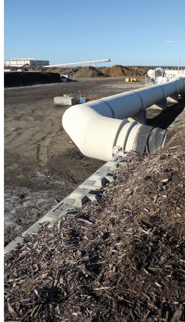
South Kern, California — aerated static pile composting with biofiltration of process air.
