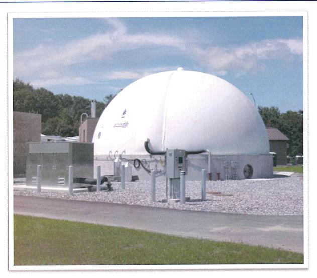
Biogas and digested sludge are stored prior to subsequent processing
