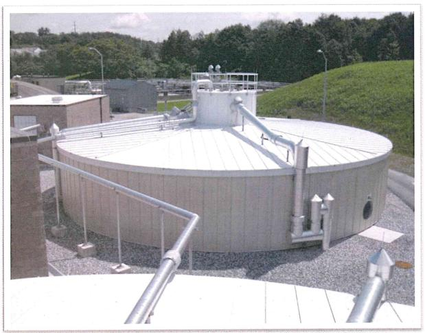
A different class of naturally present microorganisms consume organics at 95-100°F and convert a portion of the wastes to biogas
