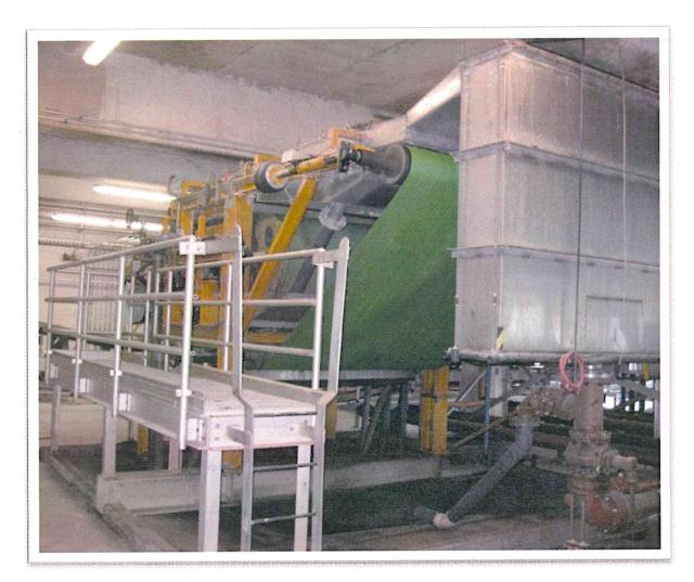
Digested sludge (aka biosolids) are dewatered using belt filter presses
