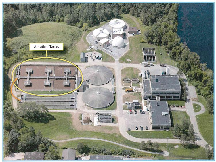
Wastewater flows to secondary treatment tanks where air is bubbled into it, allowing naturally occurring bacteria to use the waste as their food
