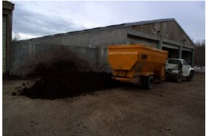
Mixing sewage sludge and sawdust for static pile composting at the Hoosac Water Quality facility in Williamstown, MA.
