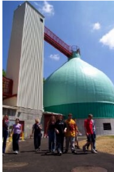
The Nashua "egg," an anaerobic digester, which produces Class B biosolids for land application, was dedicated in May, 2001. It also produces methane for energy.
