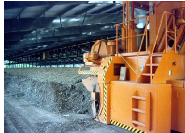
Floor aerated windrow
