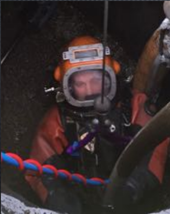
Sending a diver into a digester
