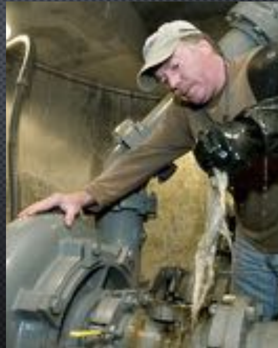
Operator removing rags and fibers from a pump
