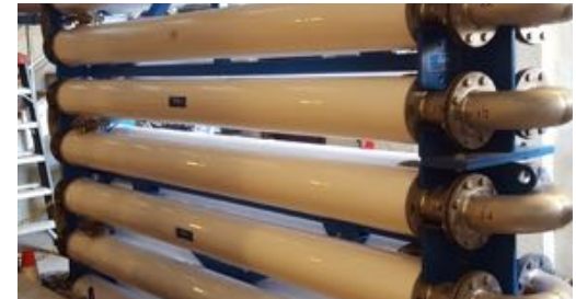
New HEX at Rockland, MA WWTP
