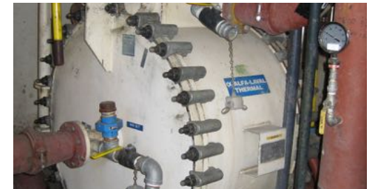
Tuning HEX for Tacoma's dual digestion process (ATAD-TPAD)
