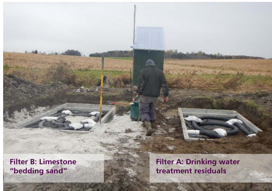
Figure 3: View of the P filters without lids and soil cover
