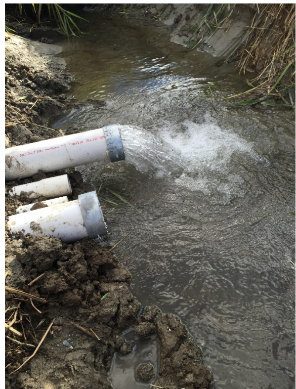
Figure 7: Filter outflow and drain pipes
