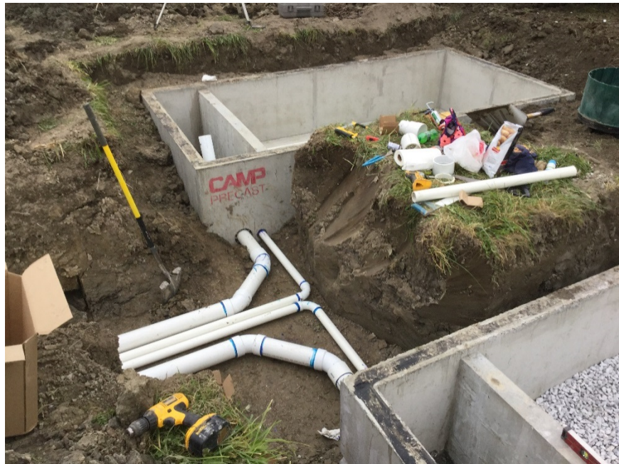
Figure 6: Constructing outflow and drain pipes
