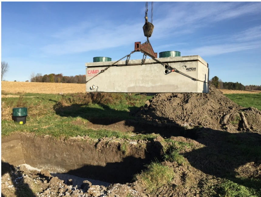
Figure 5: Placing septic tank in excavation for Filter A
