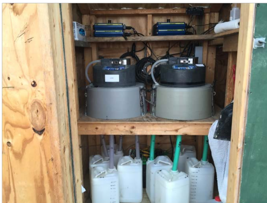
Figure 10: Autosamplers for Filter A (left) and Filter B (right) outflows
